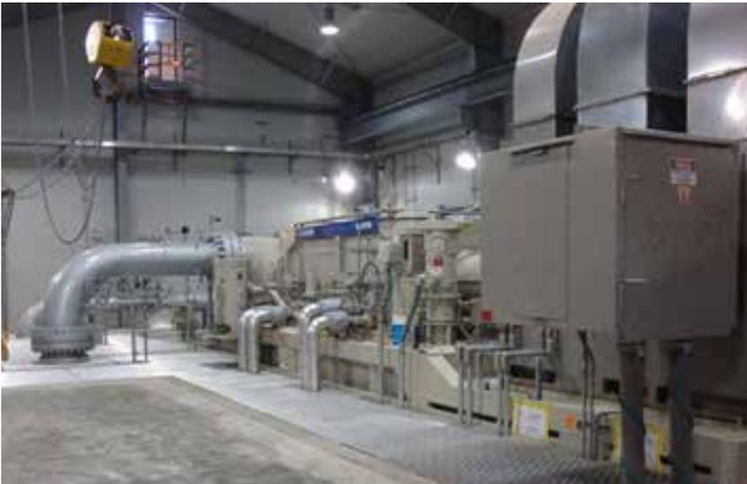
**EMD Compressor Train utilizing Voith Hydrodynamic Gearbox**
